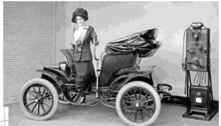
A woman with a runabout (above) with GE charger made for use in the home garage.
